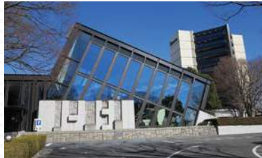
Renovation of lounge building—addition of temporary evacuation site in the case of disasters
